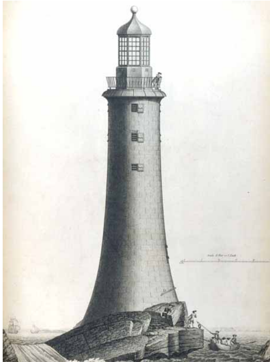
Eddystone majakas. Ajaloos esimene loodusliku hüdraulilise lubja testimine praktikas. [ http://www.lindahall.org/events_exhib/exhibit/exhibits/civil/images/eddystone_south_450.jpg ].
